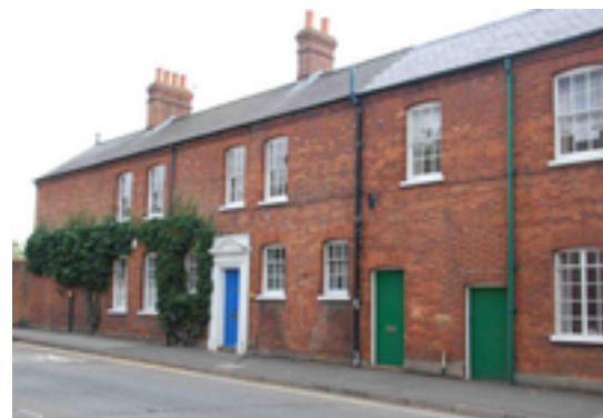
Figure 68: 1 and 3 Rectory Road
