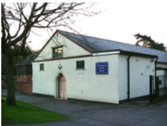
Figure 17: Masonic Centre and Malt House
