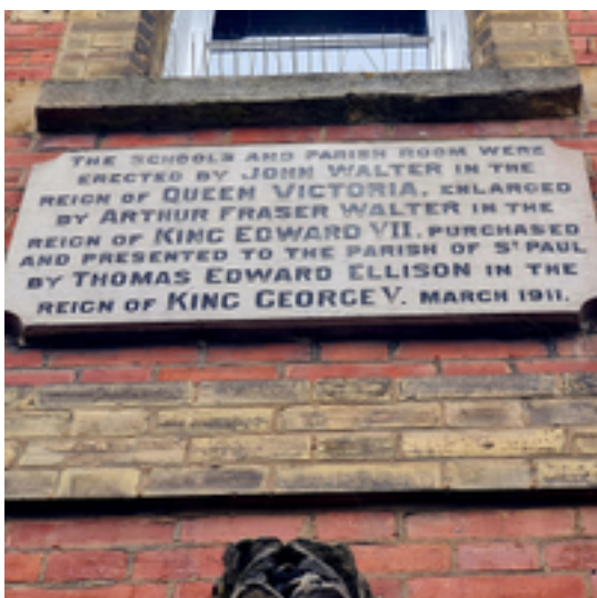
Figure 15: St Paul's Schools and Parish Room
